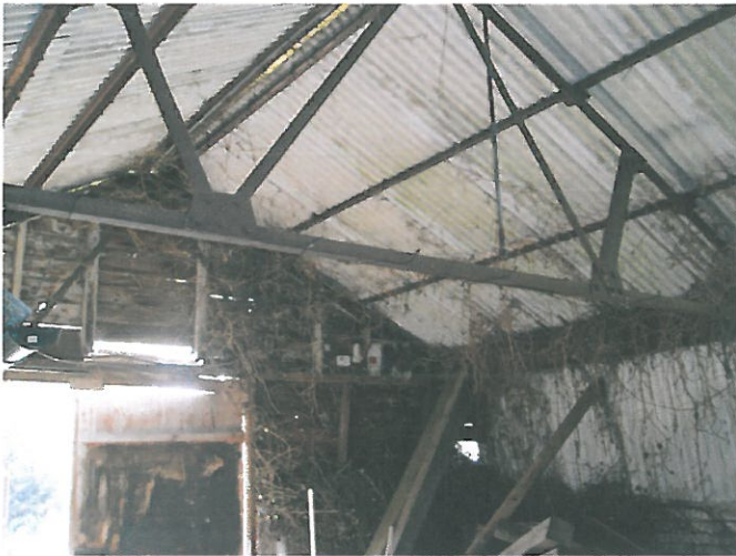
Cow Shed Steelwork
