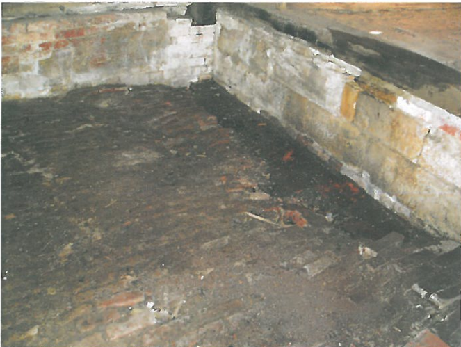
Plinth support to timber frame walls and cobbled ground floor
