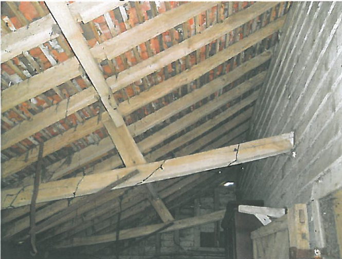
Lean to behind original Barn
